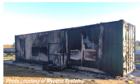
Example of damage to substation due to electrical fire
