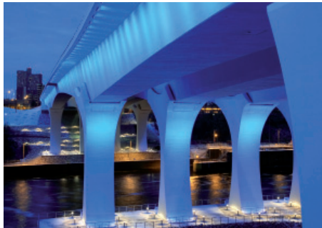
Bridge / Road Infrastructure lighting
