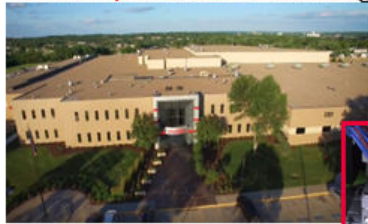
Lincoln, Nebraska Sending Plant
