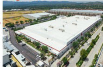
Nogales, Mexico Receiving Plant
