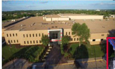
Lincoln, Nebraska Sending Plant
