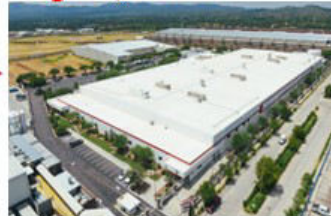
Nogales, Mexico Receiving Plant
